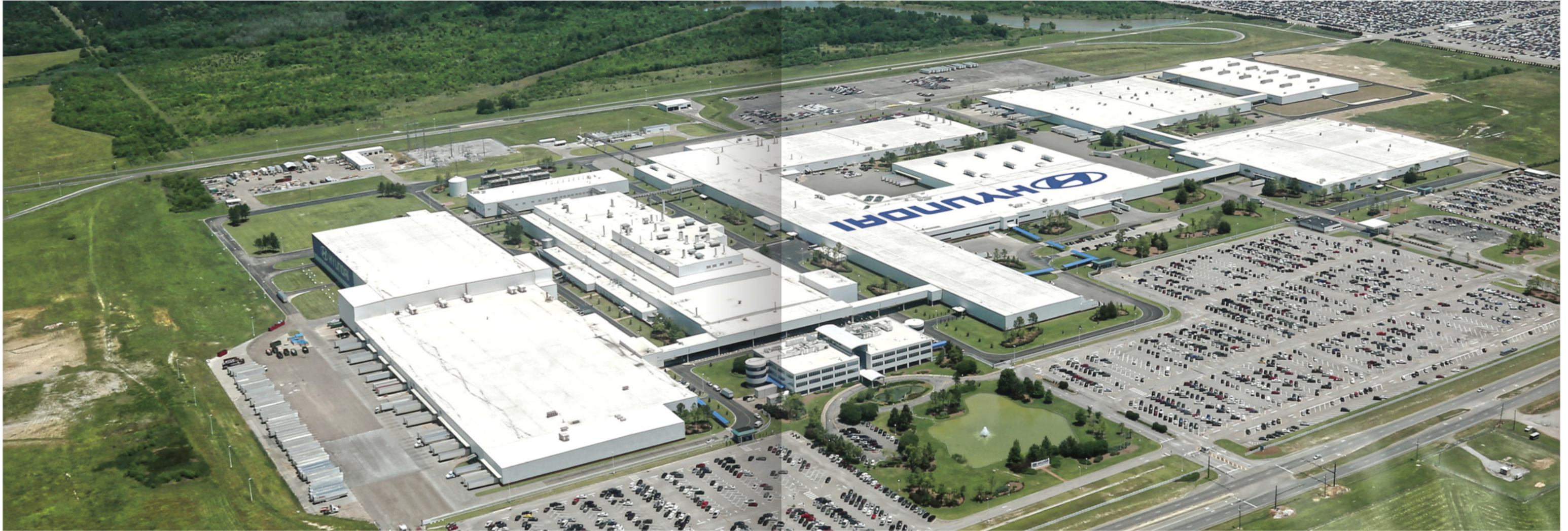
Photography 01 - Aerial view
